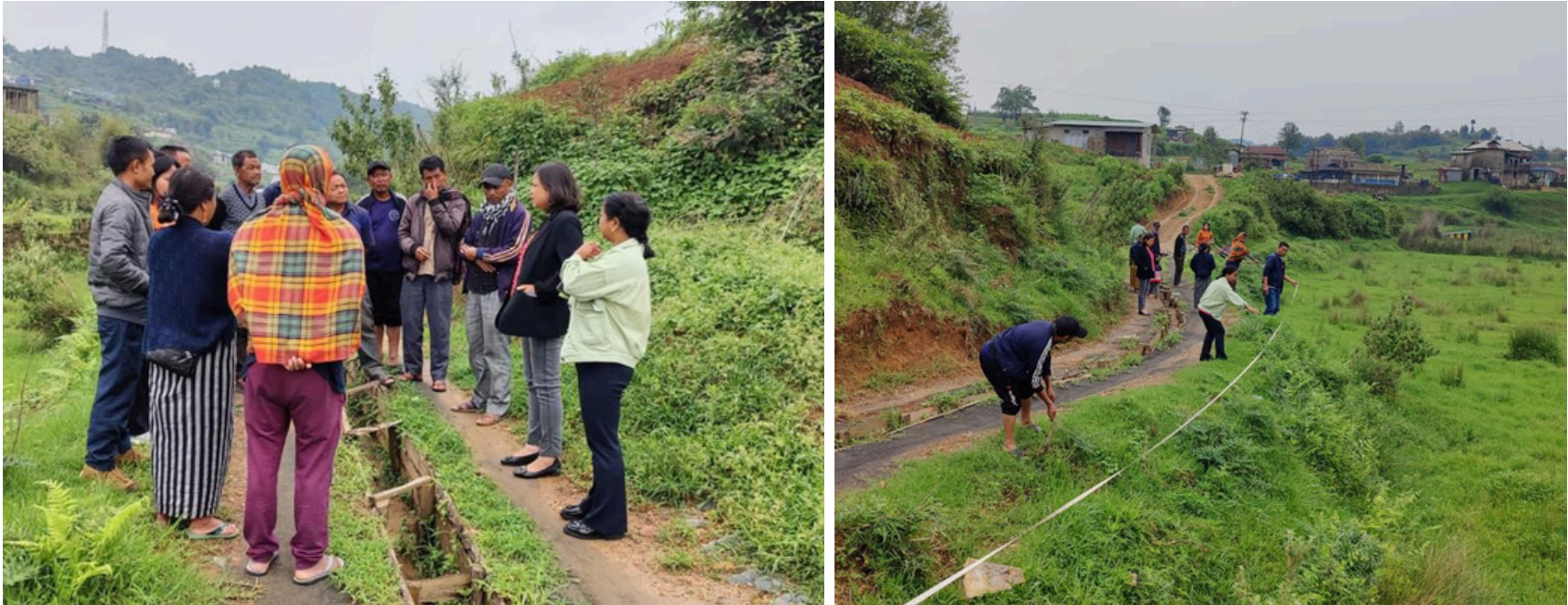
On 6th June, 2024, a site identification was conducted in the presence of Smti. A. Khongjee, DPM, EKHD, and Smti. J. Rane, A.M, BDU, along with the Executive Committee and MLAMP Committee of Lenpdengshnong, for the construction of a Protection Wall at Pamseñiong, Lenpdengshnong village under Sohiong C & RD Block.
