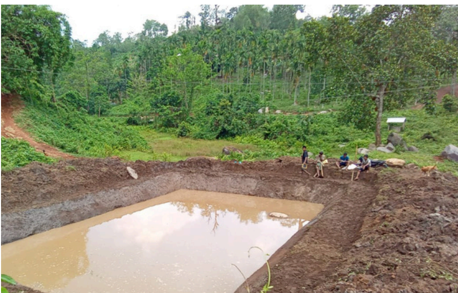
Pond excavation completed in Simseng Balkol
