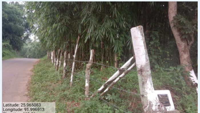
Fencing work at Nongthneng village.
