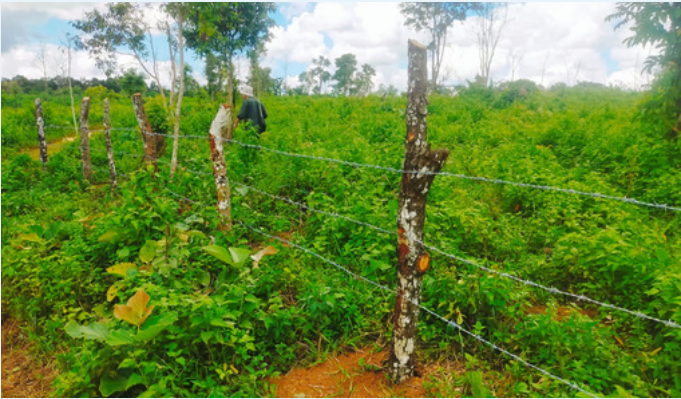
Fencing work at Umjalisiaw village.
