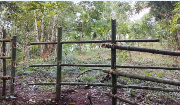
Fencing work at Lumdieng community forest.
